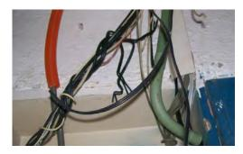
Fig. 3.2.34. Improperly joined cables and wires
