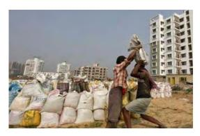
Fig. 3.1.7. Inappropriate lifting positions
