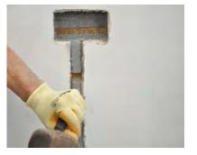
*Fig.* 7.1.2. *Chasing according to cross sectional area of conduit and switch board*
