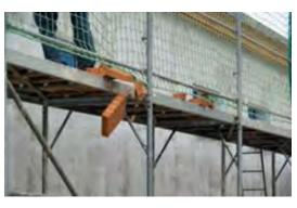
Fig. 3.1.6. Struck by an object
