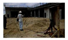
Fig. 3.2.29. Wires laying on the ground
