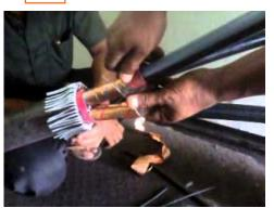
Fig. 6.1.4. joing of cables
