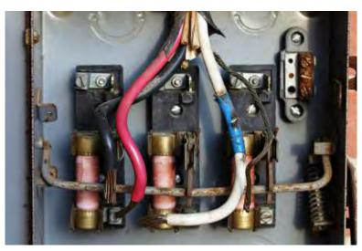
Fig. 8.2.1. Faults in Temporary Panel
