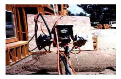
Fig. 3.2.25. Exposed switches
