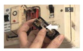
Fig. 3.2.30. Circuit breakers not turned off before use
