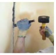
Fig. 7.1.1. Chasing on the wall with cutting tool
