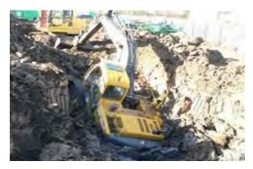
Fig. 3.1.5. Unsafe excavation
