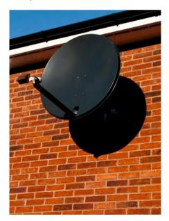
Fig 4.4.1: Wall Mount Antenna
