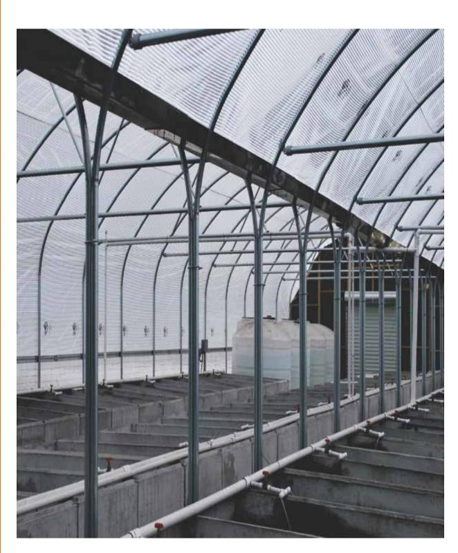
Gutter: collects and drains rain water and snow which is place at an elevated level between two spans.
