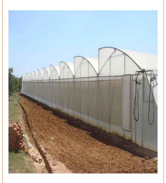
Fig 2.1.1 Saw Tooth Model
