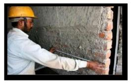
Fig-2.4.22 Measurement for vertical chasing
