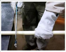
Fig-2.3.31 Pipe cutting using Hacksaws
