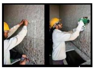
Fig-2.4.23 Chase Marking & Cutting
