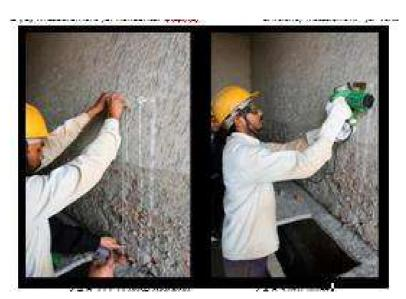
Fig-PG-0160 Chase Marking & Cutting
