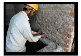
Fig-PG-0159 Measurement for vertical chasing
