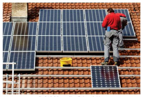
Fig. 3.1.2: Solar panel installation technicians
