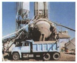
Fig 7.2.7: Transportation of concrete by trucks
