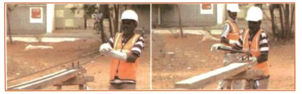
Fig 5.4.7: Bar bending by bending lever
