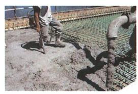
Fig 7.2.8: Placing of concrete
