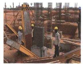
Fig 7.1.14: Dismantling of Shutter panne/s
