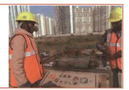
Fig 5.4.9: Bending rebar by bending machine
