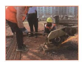
Fig 6.3.6: Cutting rebar
