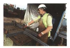
Fig 1.3.3: Bar bending work
