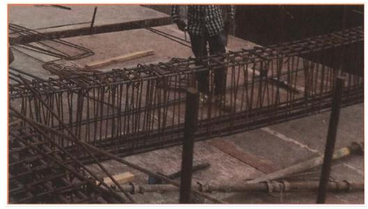
Fig. 6.2.6 Beam Reinforcement
