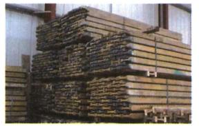
Fig 7.1.15: Storing of shutter panel
