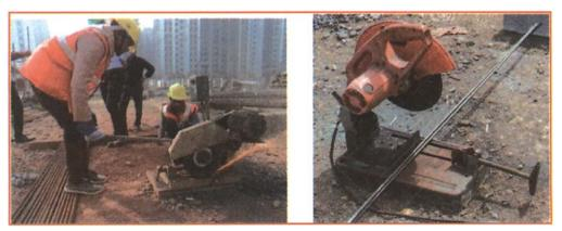
Fig 5.2.20: Cutting rebar by power saw
