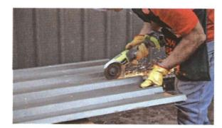
Fig 3.3.7: Cutting metal sheet
