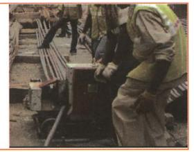
Fig 5.4.5: Cutting rebar by bar cutting machine
