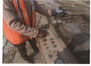
Fig 3.3.5: Rebar cutting by power saw
