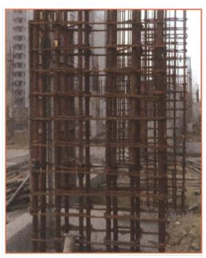
Fig. 6.2.15 Staggered lapping in column
