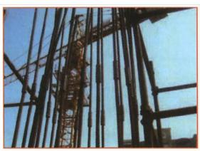
Fig 6.1.17: Mechanical lapping
