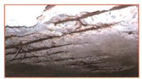
Fig 6.1.32: Effect of inadequate cover
