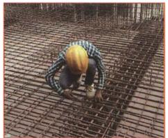
Fig. 6.2.19 Reinforcement work for slab
