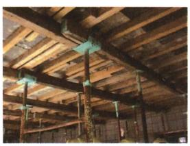
Fig 7.1.2: Conventional shuttering
