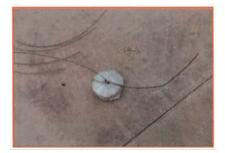
Fig 6.1.29: A typical cover blocks
