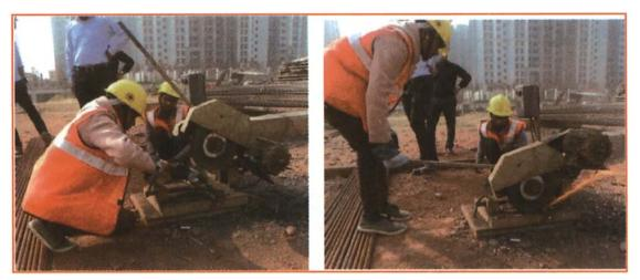
Fig 5.4.6: Cutting rebar by power saw
