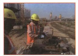
Fig 6.3.7: Bending rebar
