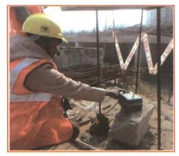
Fig 5.4.4: Operating bar cutting machine
