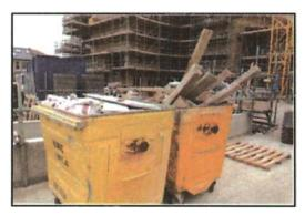
Fig 3.5.9: Segregation of construction waste
