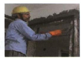
Fig 1.2.2: Plastering work
