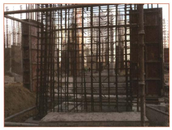
Fig. 6.2.12 Reinforcement for RCC wall
