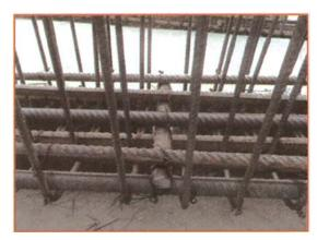
Fig 6.1.35: Rebar spacer
