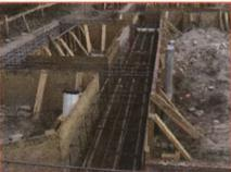
Fig. 6.2.17 Reinforcement work in beam
