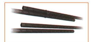
Lap splicing is done by tying the laps of rebar by wire. As we discussed in previous session, follow the procedure for tying the overlapped rebars for making the lap splice.
