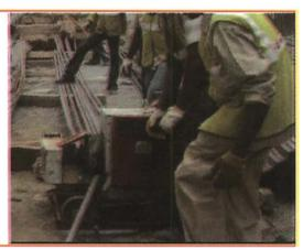
Fig 5.2.15: Cutting rebar by bar cutting machine
