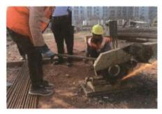
Fig 9.1.5: Rebar cutting
