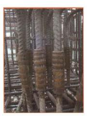
Fig 6.1.11: Rebar splicing
