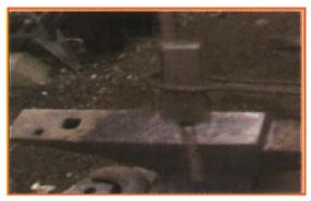
Fig 5.2.8: Cutting rebar by chisel
