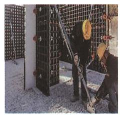
Fig 7.1.5: Steel and Aluminium in system form work
