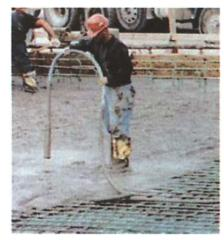
Fig 7.2.9: Compaction
