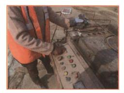
Fig 5.4.8: Operating bar bending by bending machine
