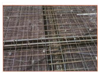
Fig 6.1.33: Concrete cover placement below rebars
