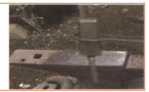
Fig 5.4.3: Cutting rebar by using hammer and chisel
