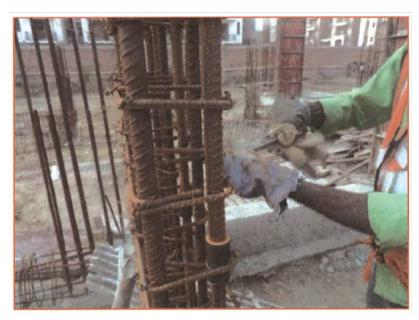
Fig. 6.2.16 Reinforcement work on column
