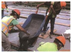
Fig 7.2.6: Transportation of concrete on wheel barrow
