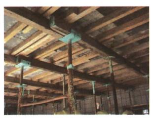
Fig 7.1.4: Timber in conventional form work
