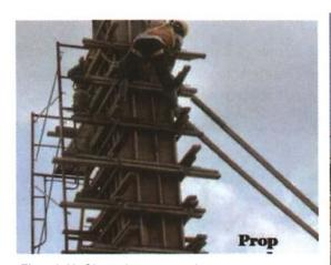
Fig 7.1.11: Shuttering prop angle
