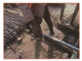
Fig 6.3.5: Marking of cutting Length
