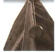
Fig 7.1.10: Plumb checking of column
