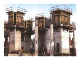
Fig 7.1.3: System shuttering
