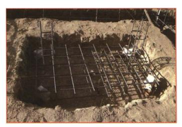
Fig. 6.2.14 Reinforcement for isolated footing
