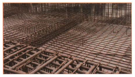
Fig. 6.2.10 Reinforcement for Slab
