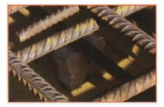
Fig 6.1.30: Placement of cover blocks
