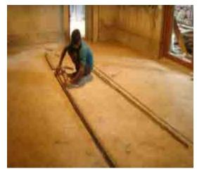
Fig. 5.2.1. Straightening of Brass/Glass strip
