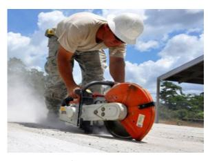
Fig. 4.2.11. Cutting concrete using Concrete Saw
