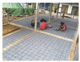
Fig. 5.1.11 Rebar used for reinforcement
