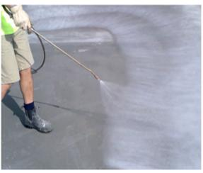
Fig. 1.3.10. Curing Concrete by water spray
