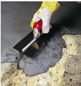
Fig.4.5.5. Spreading the mix evenly over the area to be repaired.
