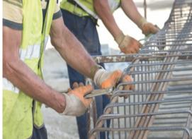
Fig. 4.3.14. Binding of Rebars
