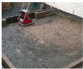
Fig. 5.1.5 Ramming of Subbase
