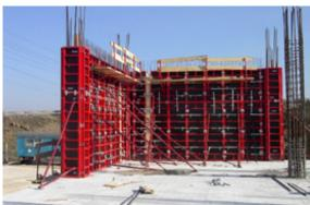
Fig. 1.2.13. Conventional formwork
