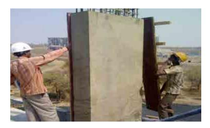
Fig. 4.3.18. Removal of Formwork
