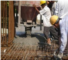
Fig. 4.1.18. Pouring of Concrete by tower crane
