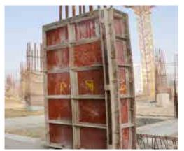
Fig. 4.3.3. Steel formwork
