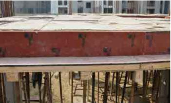
Fig. 4.3.8. Slab formwork
