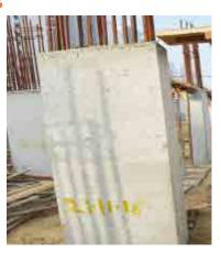
Fig. 4.3.25. Cured concrete Column
