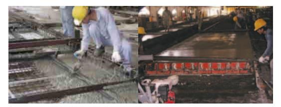
Fig.4.4.15. Screeding of poured Concrete
