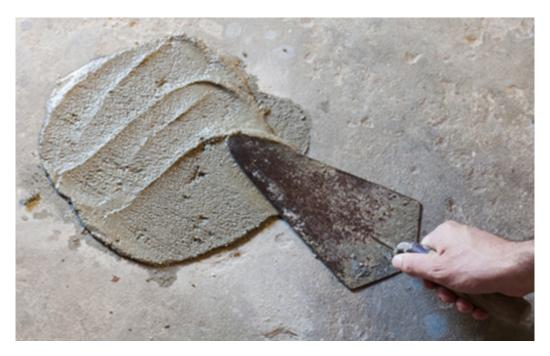
Fig.4.5.4. Applying the mix over the area to be repaired
