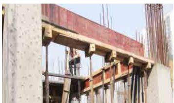
Fig. 4.3.9. Beam formwork
