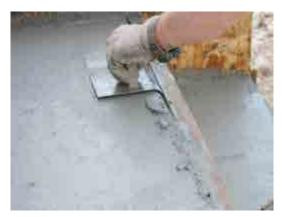
Fig. 4.1.22. Finishing concrete using edging trowel
