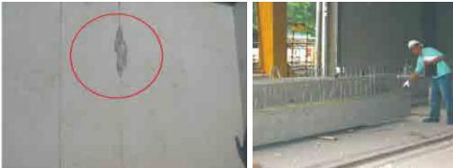
Fig.4.4.16. Inspecting the precast structure for defects and measurement corrections
