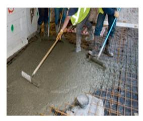
Fig. 1.3.7. Spreading Concrete
