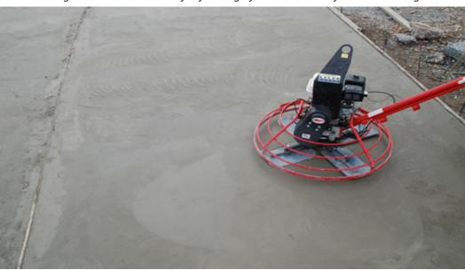
Fig. 5.3.7. Power trowel for trowelling of hardened concrete for smooth finish
