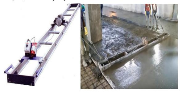
Fig. 4.2.5. Double Beam Screed Vibrator
