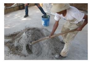
Fig. 4.1.11. Winch Machine for Concrete Mixing Fig. 4.1.12. Manual Concrete Mixing
