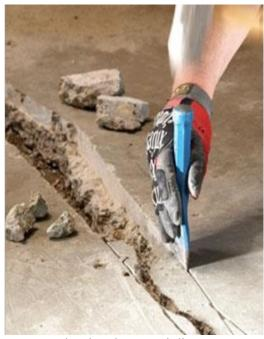
Fig.4.5.3. Chipping tools and chipping using a chisel and power drill
