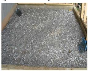
Fig. 5.1.4 Open grade stone used as Subbase
