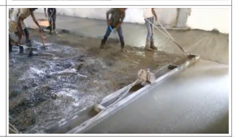
3. Compacting using double beam vibrator
