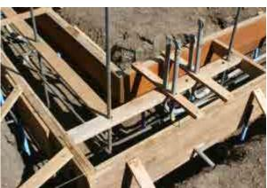
Fig. 4.3.6. Foundation formwork
