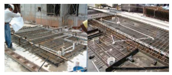
Fig.4.4.13. Inspecting the Mould before concreting
