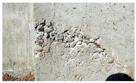
Fig.4.5.1. Defect in concrete structure due to honeycombing
