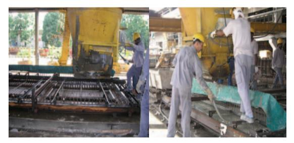
Fig.4.4.14. Pouring concrete in the Mould and compacting
