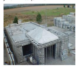
Fig. 4.3.4. Aluminium formwork
