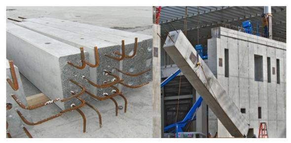
Fig.4.4.7. Precast Concrete Columns
