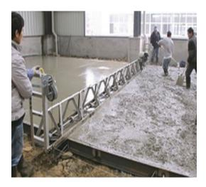
Fig. 1.3.9. Screeding of Concrete
