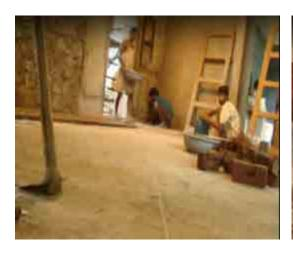
Fig. 5.2.3. Positioning of Brass/Glass strip
