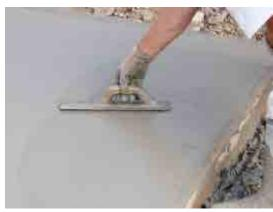
Fig. 4.1.23. Finishing concrete using concrete trowel
