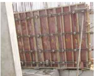
Fig. 4.3.7. Wall formwork
