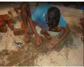
Fig. 5.2.4. Laying of Brass/Glass strip
