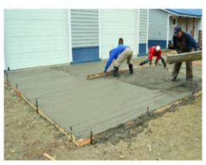
Fig. 5.2.6. Placing of Concrete
