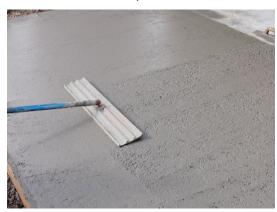
Fig. 4.1.21. Finishing concrete using bull float
