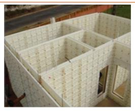
Fig. 4.3.5. Plastic formwork
