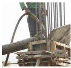
Fig. 4.3.21. Pouring & Compacting
