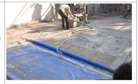
7. De-watering using the vacuum de-watering system
