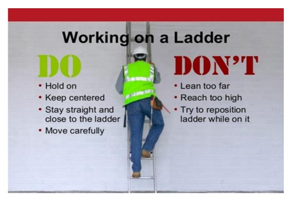
Fig. 3.2.10. Safety Rules for using Ladder
