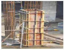
Fig. 4.3.20. Formwork
