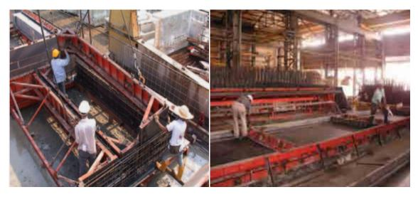
Fig.4.4.8. Assembling Mould
