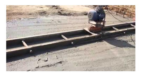
Fig. 5.1.13 Compacting using double beam screed vibrator
