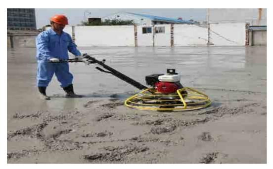
Fig. 5.3.6. Power trowel for floating of wet concrete after de-watering
