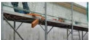
Fig. 3.1.5. Risk of Falling of Debris
