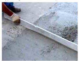
Fig. 4.1.20. Striking off concrete using straight edge
