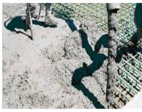
Fig. 1.3.8. Compacting Concrete using Vibrator
