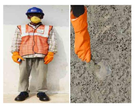
Fig. 3.2.7. personal protective equipments while concreting
