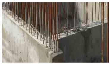
Fig. 4.3.40. Concrete foundation after Deshuttering
