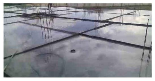
Fig. 4.1.24. Curing of concrete using water
