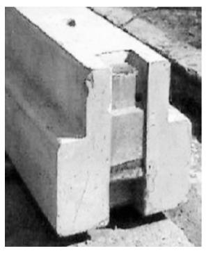
Fig.4.4.5. Inverted T Beam
