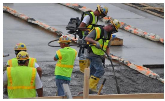
Fig. 3.2.6. personal protective equipments while using needle vibrator
