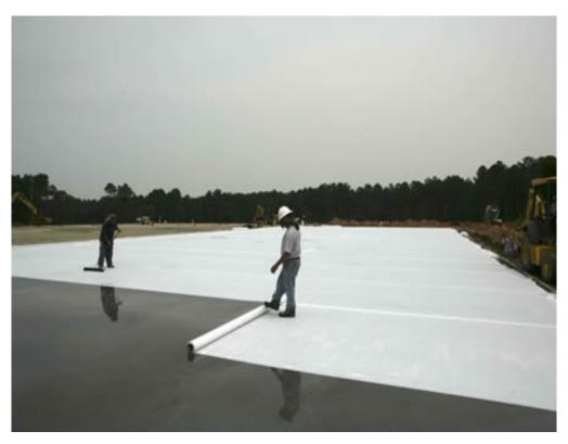
Fig. 4.1.25. Curing using plastic membrane
