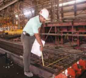
Fig.4.4.10. Adding Rebars to the Mould
