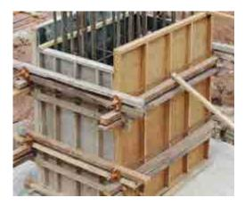
Fig. 4.3.1. Plywood formwork
