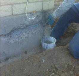
Fig.4.5.7. Repairing defects in the foundation
