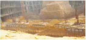
Fig. 3.1.7. Unsafe Excavation without Barricading
