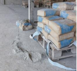
Fig. 4.1.6. Right way of Stacking Cement
