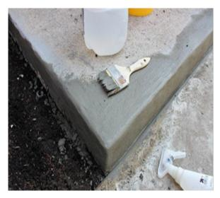
Fig.4.5.6. Repaired floor corner
