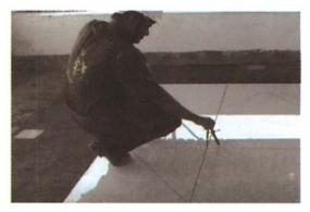
Fig 8.1.5: Marking on tiles
