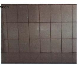
Fig 6.1.6: Checking for excessive grout on wall
