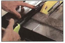
Fig 5.2.10: Positioning tile on the wet saw
