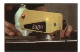
Fig 5.2.12: Cutting Tile by wet saw
