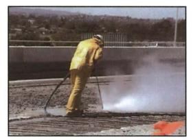
Fig 5.3.2: High pressure water blasting
