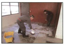
Fig 5.3.3: Acid etching
