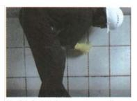
Fig 6.1.5: Wiping grout on wall
