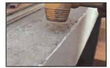
Fig 5.3.31: Inserting dowels in surface
