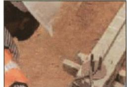
Fig 1.2.4: Bar bending
