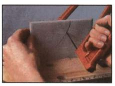
Fig 5.2.6: Cutting curves on tile
