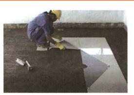
Fig 8.1.7: Placing a/tiles
