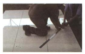
Fig 8.1.4: Measuring & marking on tiles
