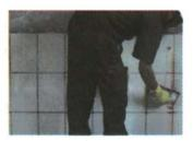
Fig 6.1.4: Applying grout on joints
