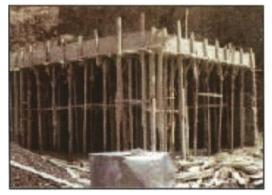
Fig 1.2.5: Conventional formwork
