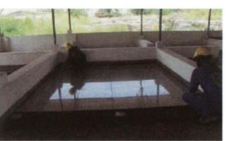
Fig 1.3.1: Placing tiles on the surface
