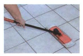
Fig 6.2.2: Mopping after curing of grout
