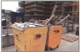
Fig 3.5.9: Segregation of construction waste
