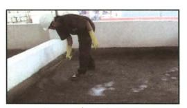
Fig 5.3.1: Cleaning surface by broom
