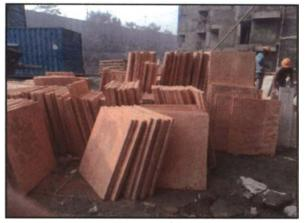
Fig 4.2.14: Storing and stacking a/tiles
