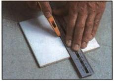
Fig 5.2.3: Marking on tile by steel rule
