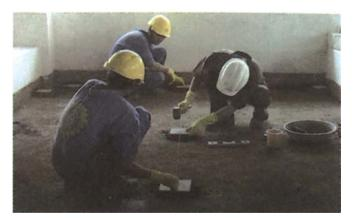
Fig 8.2.2: Levelling of butter mark
