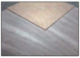
Fig 5.3.24: Placing first tile for reference
