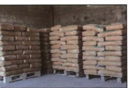
Fig 4.2.12: Stacking of cement bags
