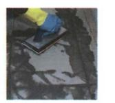
Fig 6.1.3: Applying grout on joints
