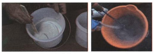
Fig 6.1.1: Stirring grout by stirrer or hand held mixer
